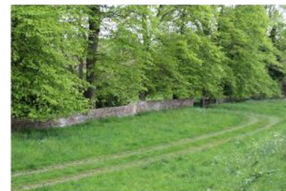
P. Vantage point: Trinity House, Cambridge Rd, Gt Shelford View: looking SW to WSW over pasture at Trinity House & open arable land
