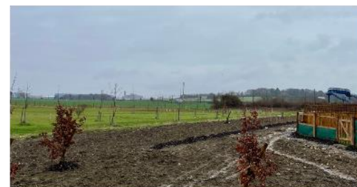
Q. Vantage point: More's Meadow, Gt Shelford (construction ongoing in foreground) View: scanning N to NE across open arable fields & railway towards Nine Wells & White Hill
