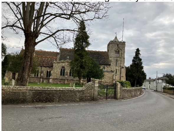
Fig 3.7.1 View south along Church Lane
