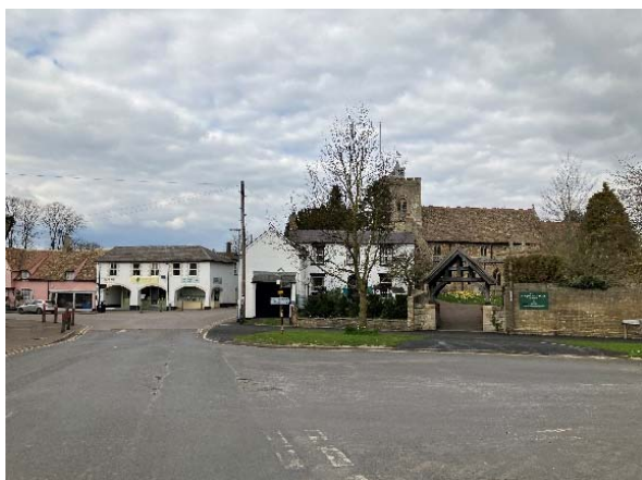
Fig 3.7.3 View north on School Ln to High St
