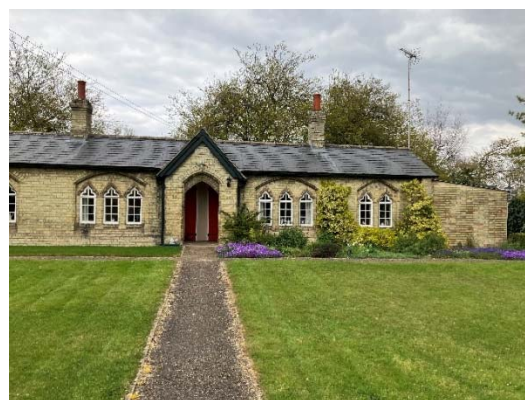
Fig 4.3.1 Alms Houses, Church Lane, Fulbourn
