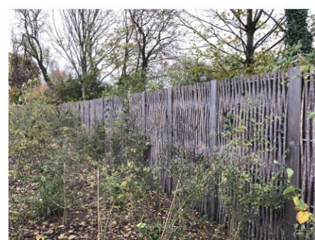
Precedent image of Fencing interface: woven willow acoustic fencing at Cambridge North Station
