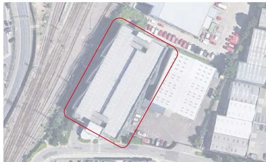
Cambridge Leisure Park Car Park
