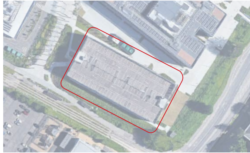
Cambridge Science Park Multi-storey Car park
