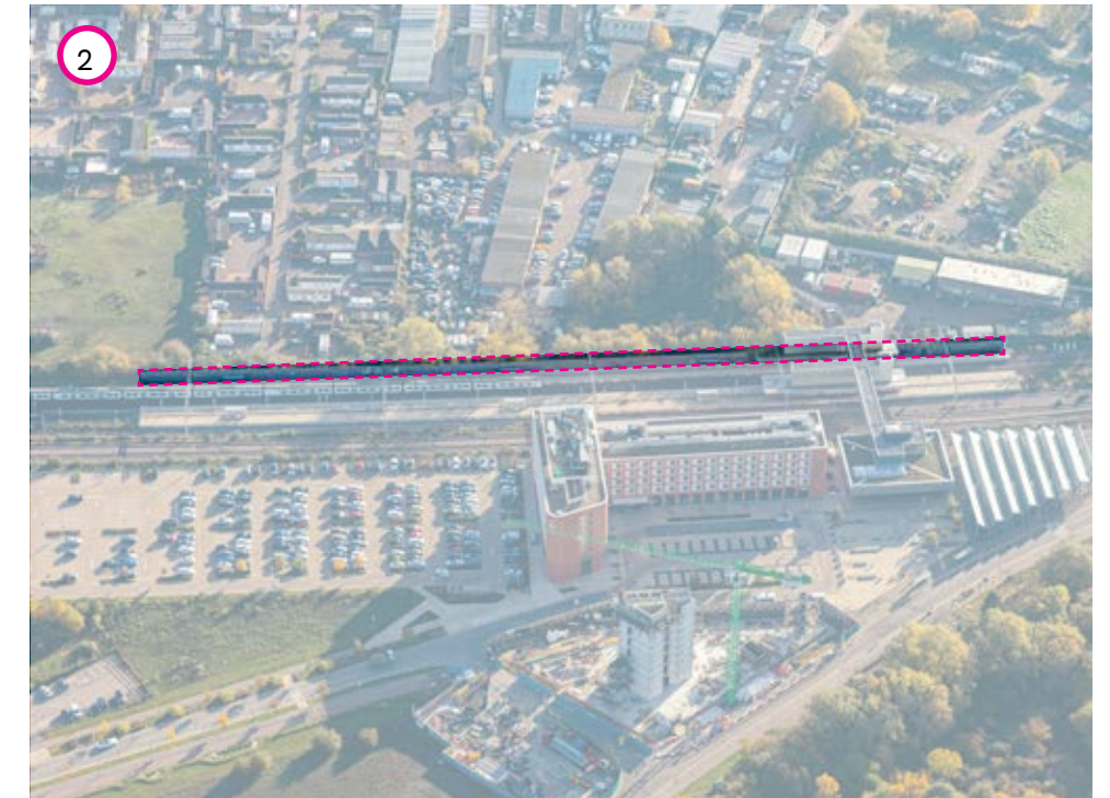
2 - Existing sound barrier east of tracks
