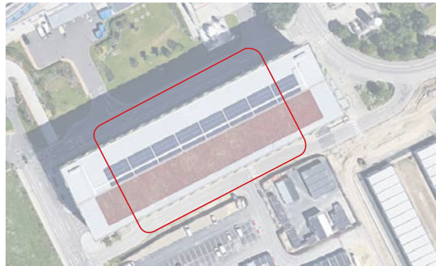
Cambridge Addenbrooke Multi-storey Car park
