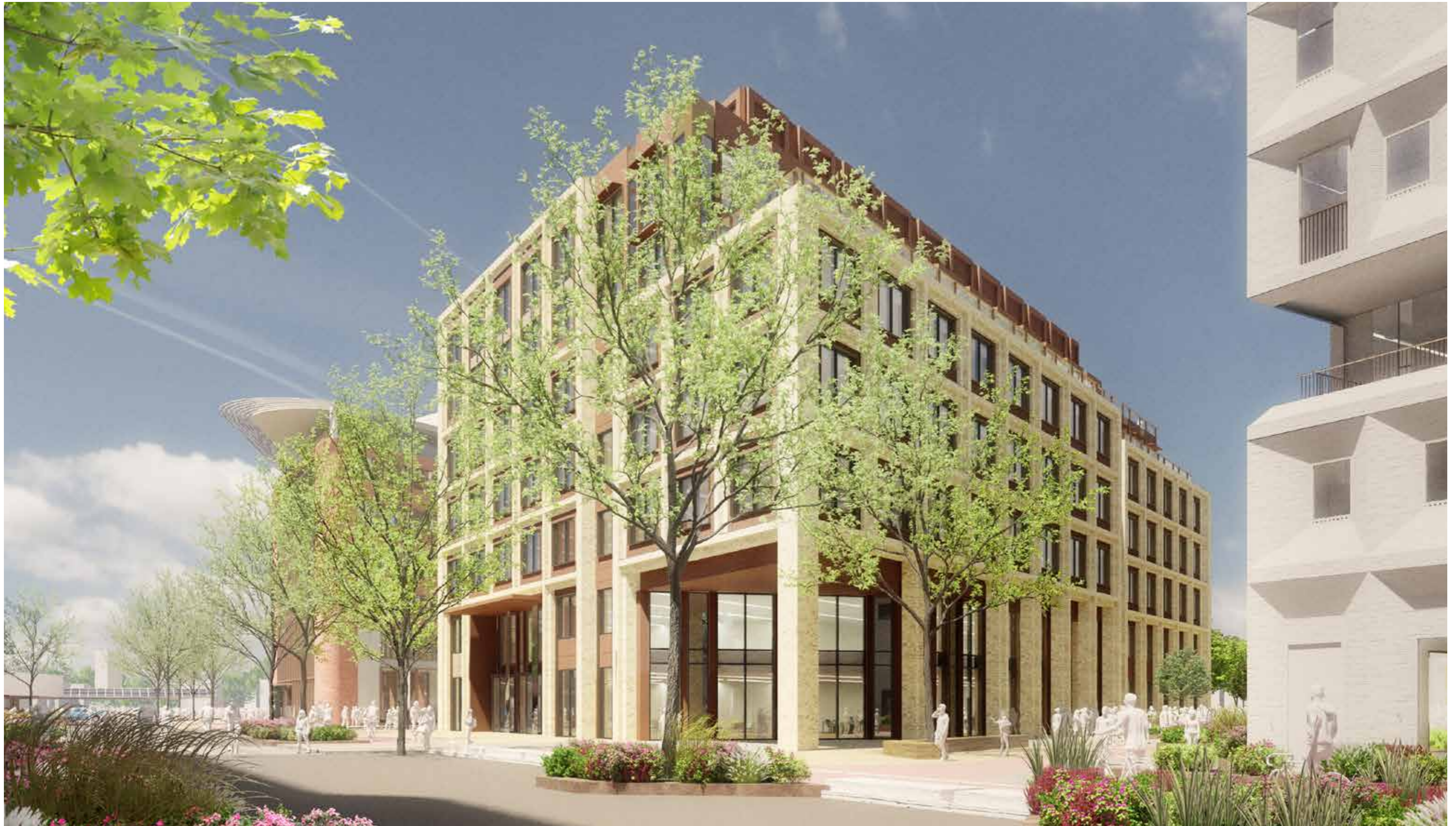
Illustrative view of One Milton Avenue from the north-east at the junction of Milton Avenue and Milton Walk.
