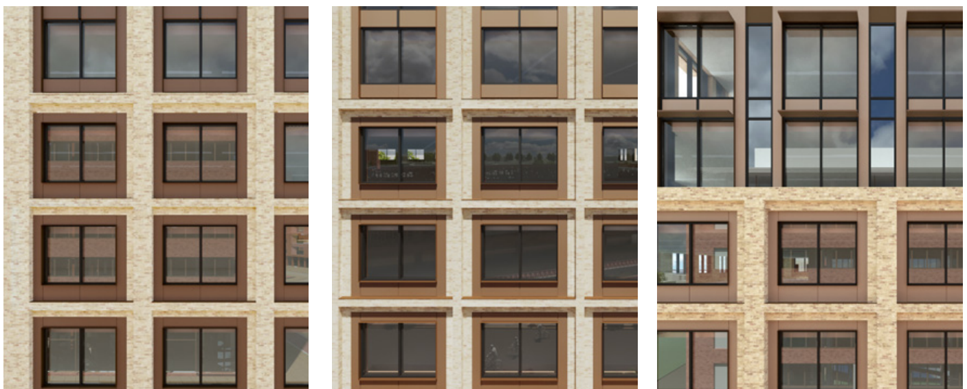
Fig. 21 Facade depths and articulation respond to orientation, maximise shading and minimise solar gain.
