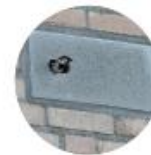
Bird house on facade
