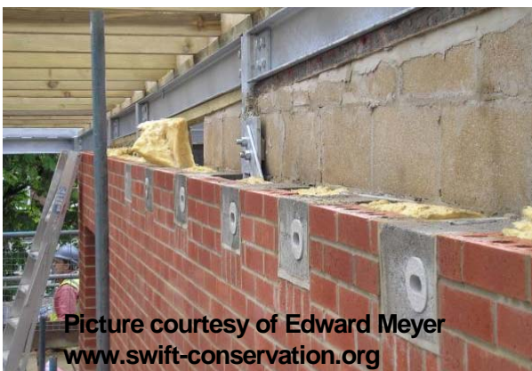
Many specialist nest and bat boxes can be purchased. These swift brick-boxes are being built-in to dwellings in New Barnet for the Notting Hill Housing Trust.
