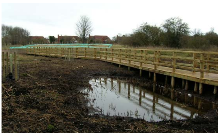
Stockbridge Meadows Riverside Park has been provided by Manor Kingdom Ltd for Melbourn Parish Council through a legal agreement attached to a planning decision.
