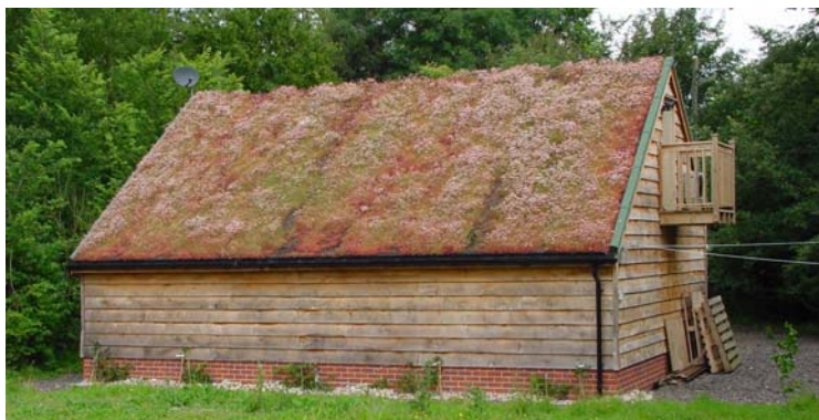
A private building using green roof techniques to lessen the visual impact.
