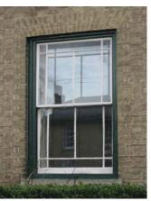
(left) Horizontal sliding (Yorkshire) sash window (middle) Side opening casement window (right) Vertical sliding sash window (with circa 1800 marginal light design)
