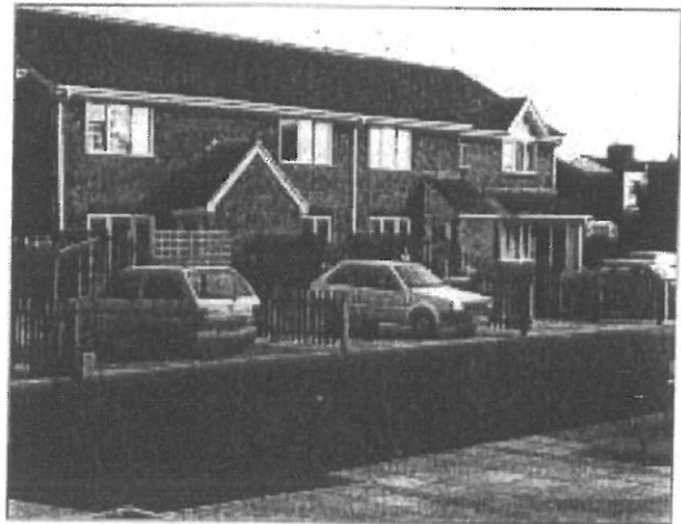
High parking standards reduce the frontage available for landscaping
