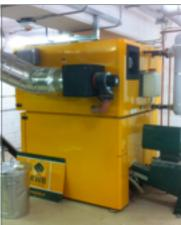
Photo I: Front elevation and biomass boiler, Richard Newcombe Court, Cambridge.
