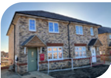
New Council homes under construction in Cottenham
