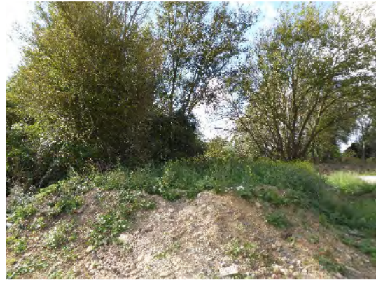
Photograph 10: Earth mound along the south of the barrel-field
