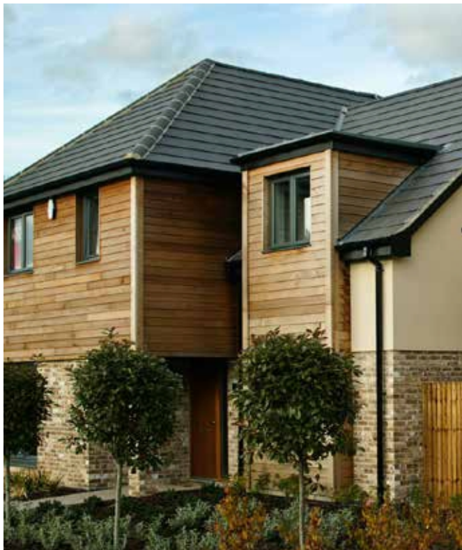
Figure 26: Histon Housing, R H Partnership Architects
