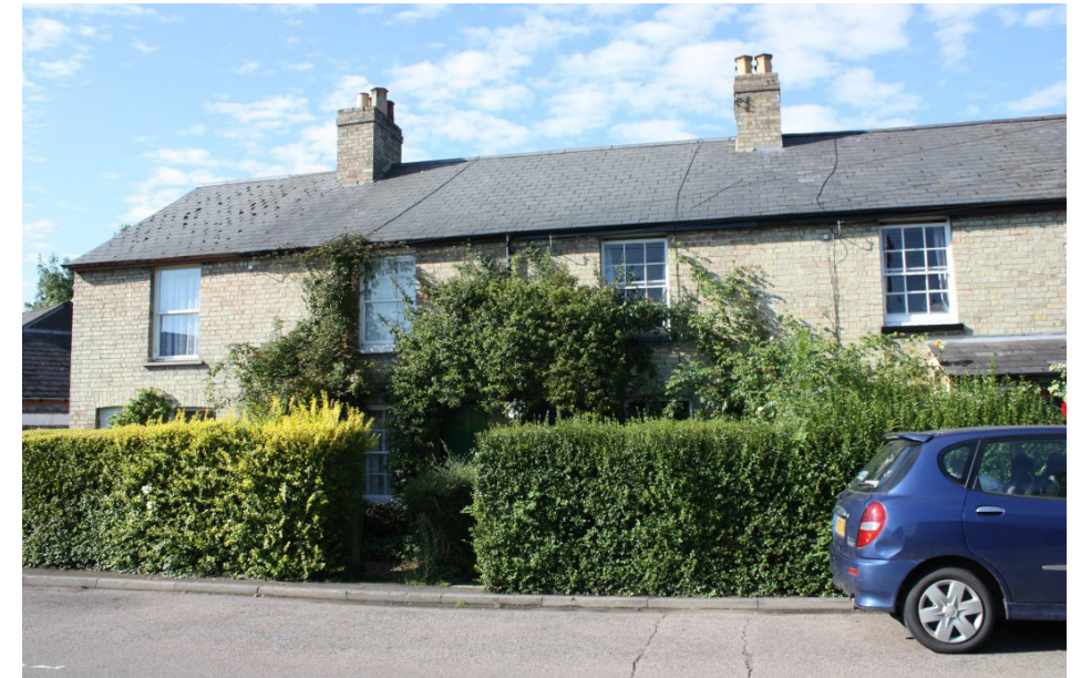
Figure 51: Victorian Terrace, 21-27 Hauxton Road
