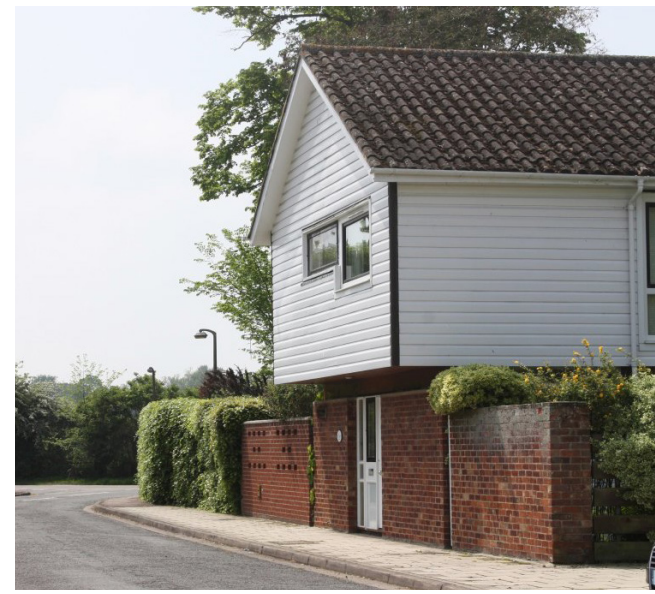
Figure 18: 1 Courtyards, Whittlesford Road
