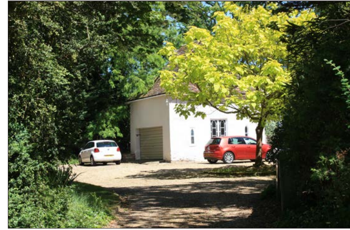
Figure 70: Kings Farmhouse Dovecote, 21 High Street.
