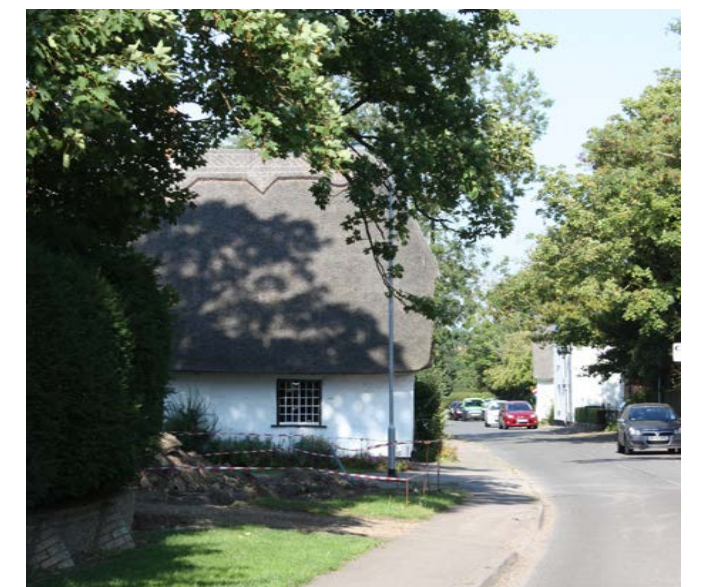
Figure 26: White's Farm House, 26 High Street
