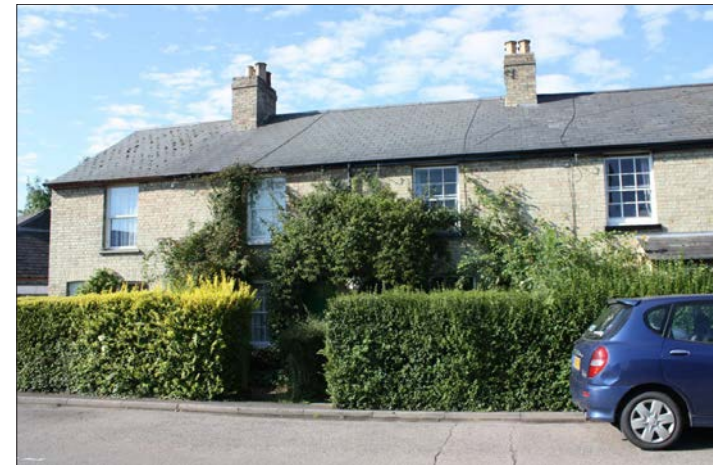
Figure 67: Terrace, 21-27 Hauxton Road.
