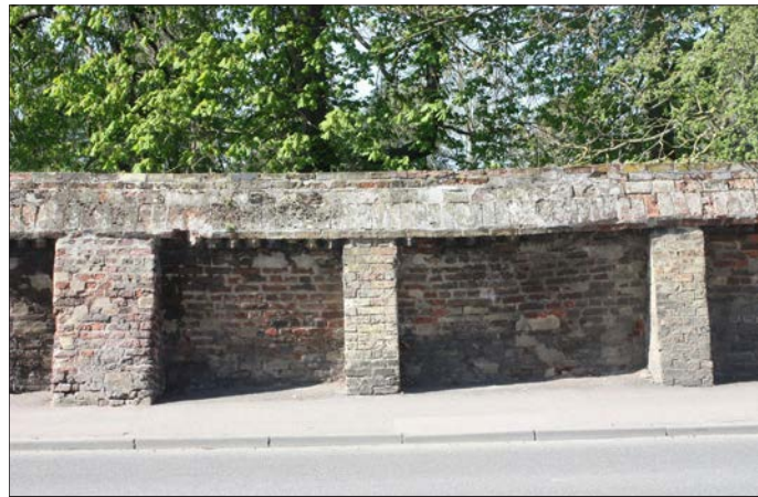
Figure 75: Boundary wall. The Manor House, Bridge Lane.
