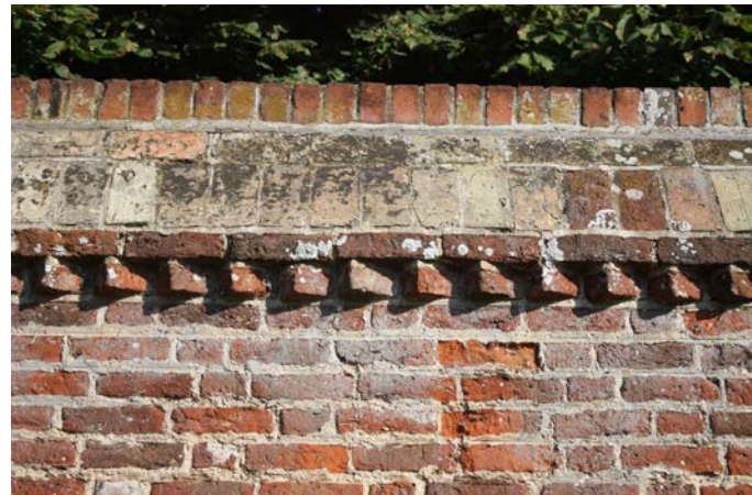
Figure 77: Boundary wall. The Manor House, Bridge Lane.
