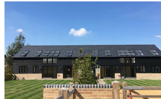
Figure 106: Terraced housing in Haslingfield
