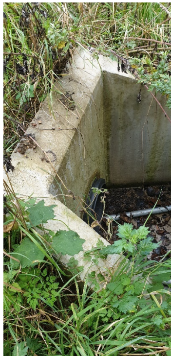
Photograph 5.11: Overflow pipe of the Kingfisher Pond, October 2020
